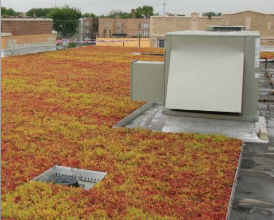
Roof with Exposed Membrane
