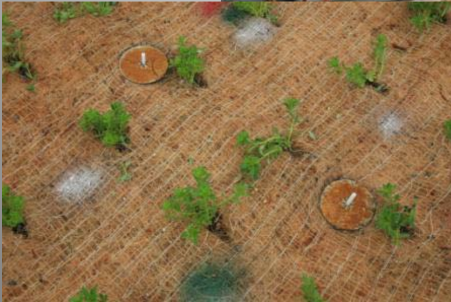
Erosion control matting Chicago, IL
