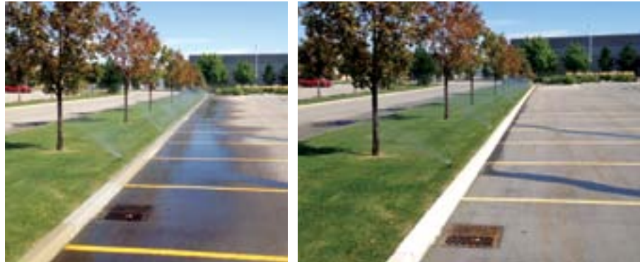
Water was being wasted with overspray (left), but with improvements, both water and energy are conserved.
