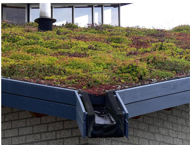
A green roof typically incorporates a high-quality waterproofing and root repellent system, a drainage system, filter cloth, a lightweight growing medium, and the plants themselves. Green roofs can also complement man-made “grey” infrastructure by absorbing rainwater polluted runoff and can also mitigate urban heat island effect.<sup>72</sup> During the summer months, green roofs can retain 70-90% of precipitation that falls and, in winter months, can absorb 25-40% of snowfall.<sup>73</sup>
