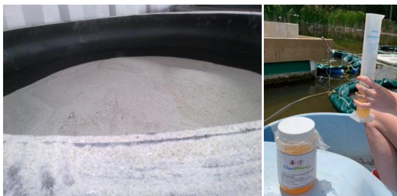
Figure 4. Wollastonite crystals in pilot treatment system cell (L), and ClariPhos™ being dosed into a treatment mesocosm (R).
